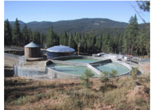
A slow sand filter system
